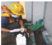
Location Plant room
